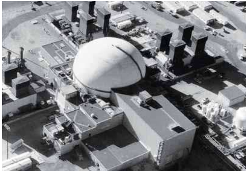
Figure 7.4 Fast Flux Test Facility at Hanford, Washington. Source: Federation of American Scientists.
