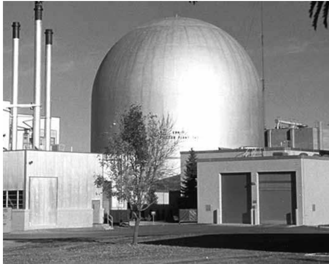
Figure 7.2 Experimental Breeder Reactor-II. Source: Argonne National Laboratory.
