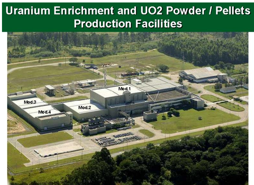
Figure 11: Layout of INB centrifuge cascade modules at Resende facilities (Source: INB – IndustriasNucleares do Brasil)
