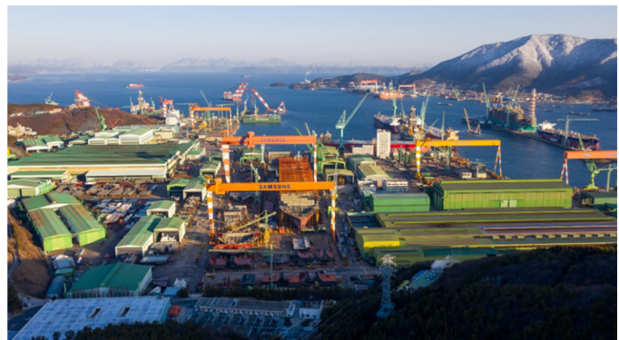
Figure 1. Modern shipyard fabrication model. The Samsung Heavy Industries Co. shipyard in Geoje, South Korea illustrates the capability and capacity of modern shipyards to fabricate the largest ships in the world—including oil tankers, container ships, and floating production, storage and offloading platforms. Photographer: SeongJoon Cho/Bloomberg via Getty Images. Used with permission.
